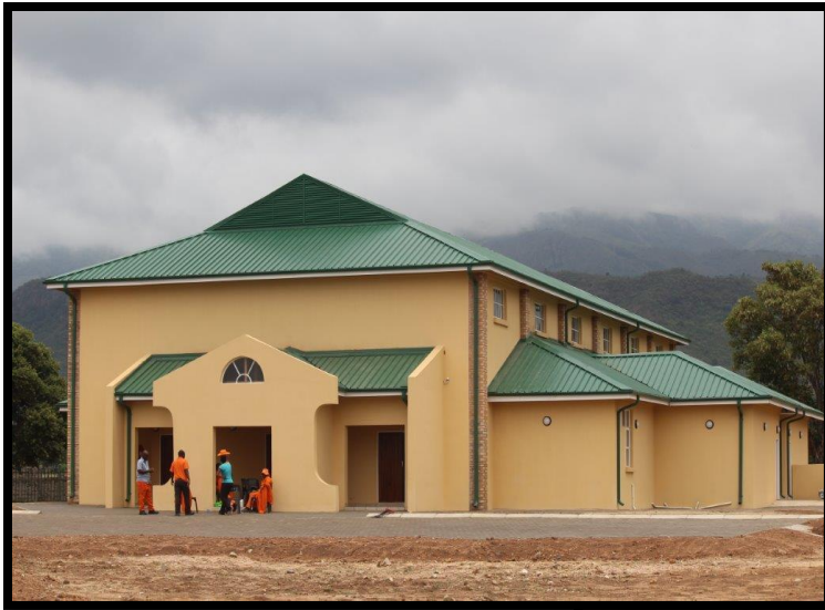
Moshate Community Hall
